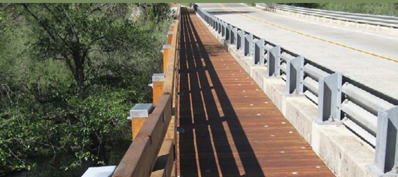
BIKE LANE BESIDE RIVER OVERPASS
